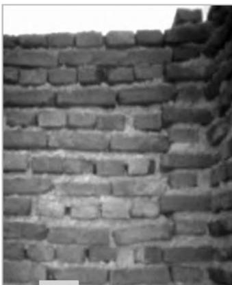
Figure 3.12: Improper bonding of masonry units
