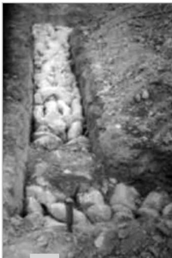
Figure 3.8: Stone Masonry in Foundation
