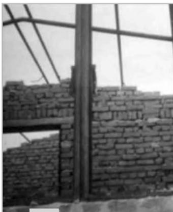
Figure 3.11: Pre Cast RCC lintel above the opening
