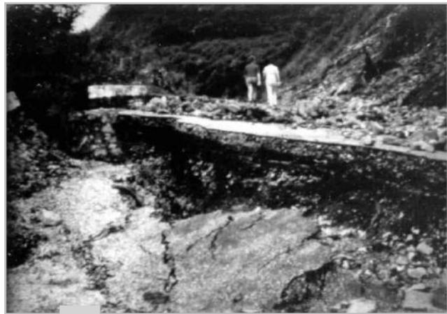
Figure 3.4: The damage of road in Koshi Highway
